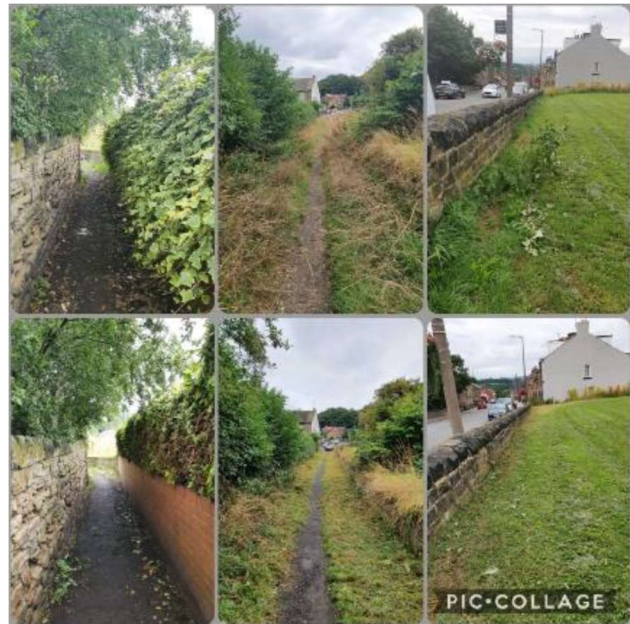
59. 05/08/2021 – Park Road Playing Field, Worsbrough Ward Widened the footpath by defining the edges. Strimmed the perimeter of the field and trimmed the hedges. Activities to be followed up during the week with volunteers.
