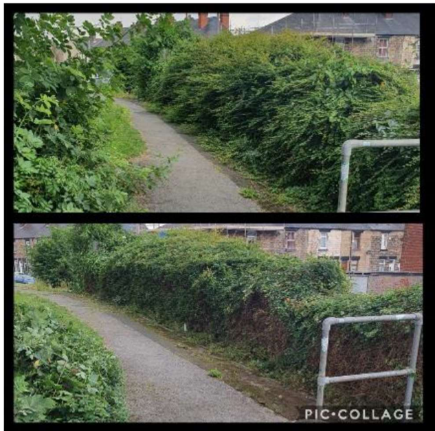
57. 04/08/2021 - Blenheim Avenue, Kingstone Ward Trimmed back the shrubs obstructing the footpath.
